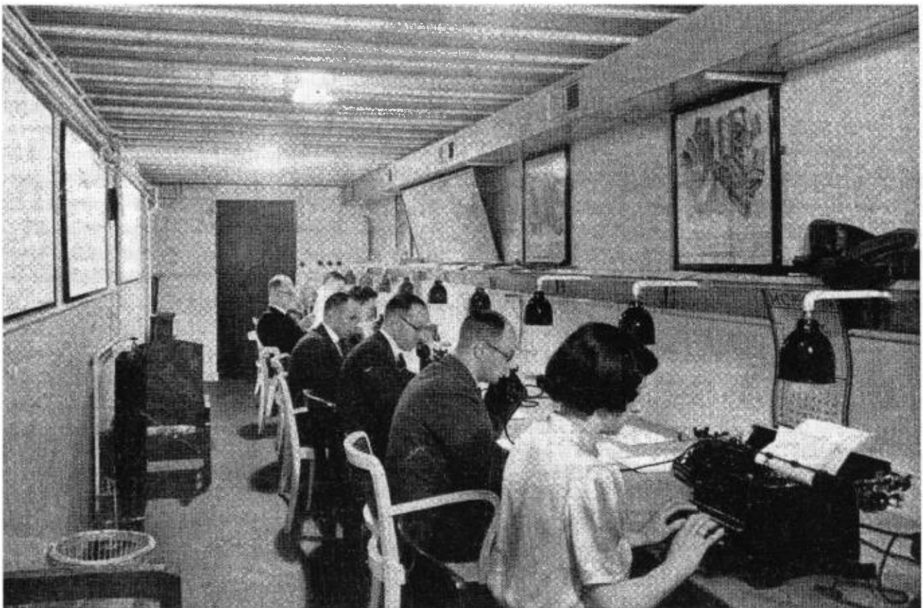
The Control Room, WW II Southern Railway Communications Bunker, Deepdene, Dorking
